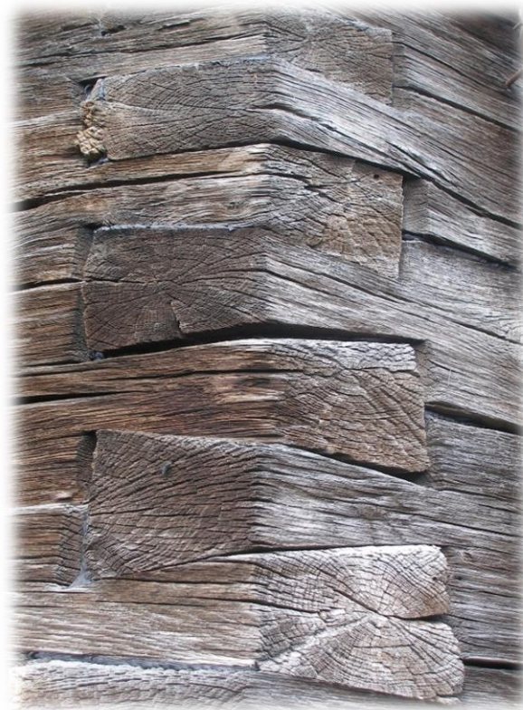
Method of building wooden churches in Turopolje - joining wooden beams
